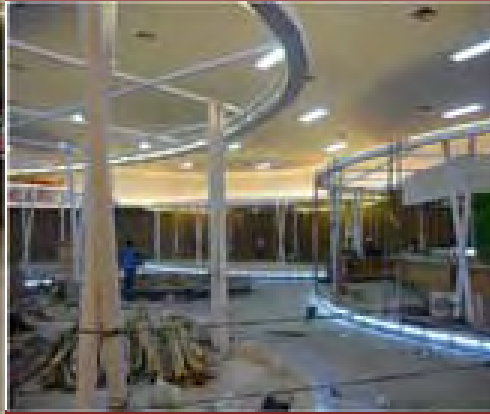
Enhancement work underway
